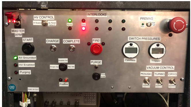
FIG. 4. Arduino Uno (ATmega328P-based) control panel for semi-autonomous control of the BLUE charging and firing sequence, as well as other system functions.
